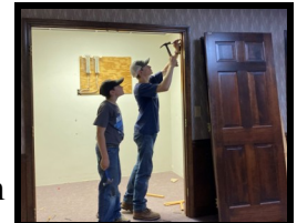
Two grandsons pulling down walls to make room for apartment dividers.
